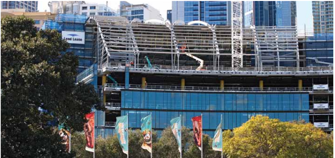
Commonwealth Bank Place under construction
