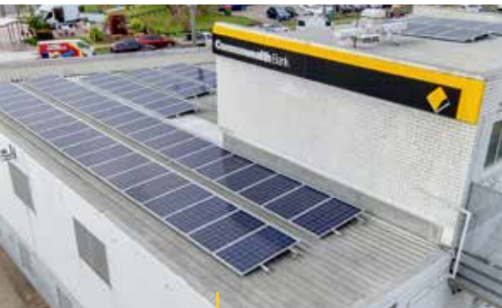
Solar panels on our branches reduce our environmental impact and our costs
